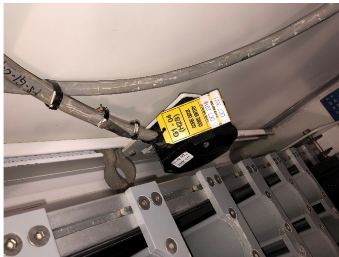
Figure 28. H2S fixed H2S monitor
