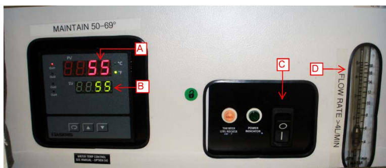
Figure 1. HASKRIS Control Panel. (A) Actual temperature. (B) Set temperature. (C) On/Off switch. (D) Flow meter.
