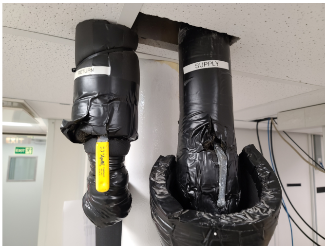
Figure 7: Ship's chill-water valves shown open.
