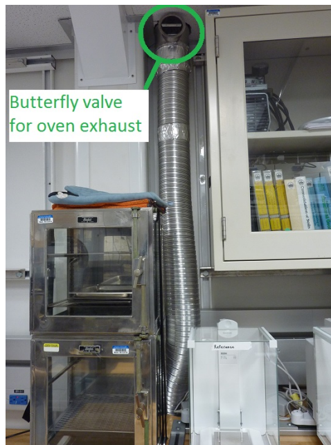
Figure 5. Exhaust tubing and butterfly valve control (green circle). The butterfly is completely closed. The desiccator boxes are to the left of the exhaust tubing.
