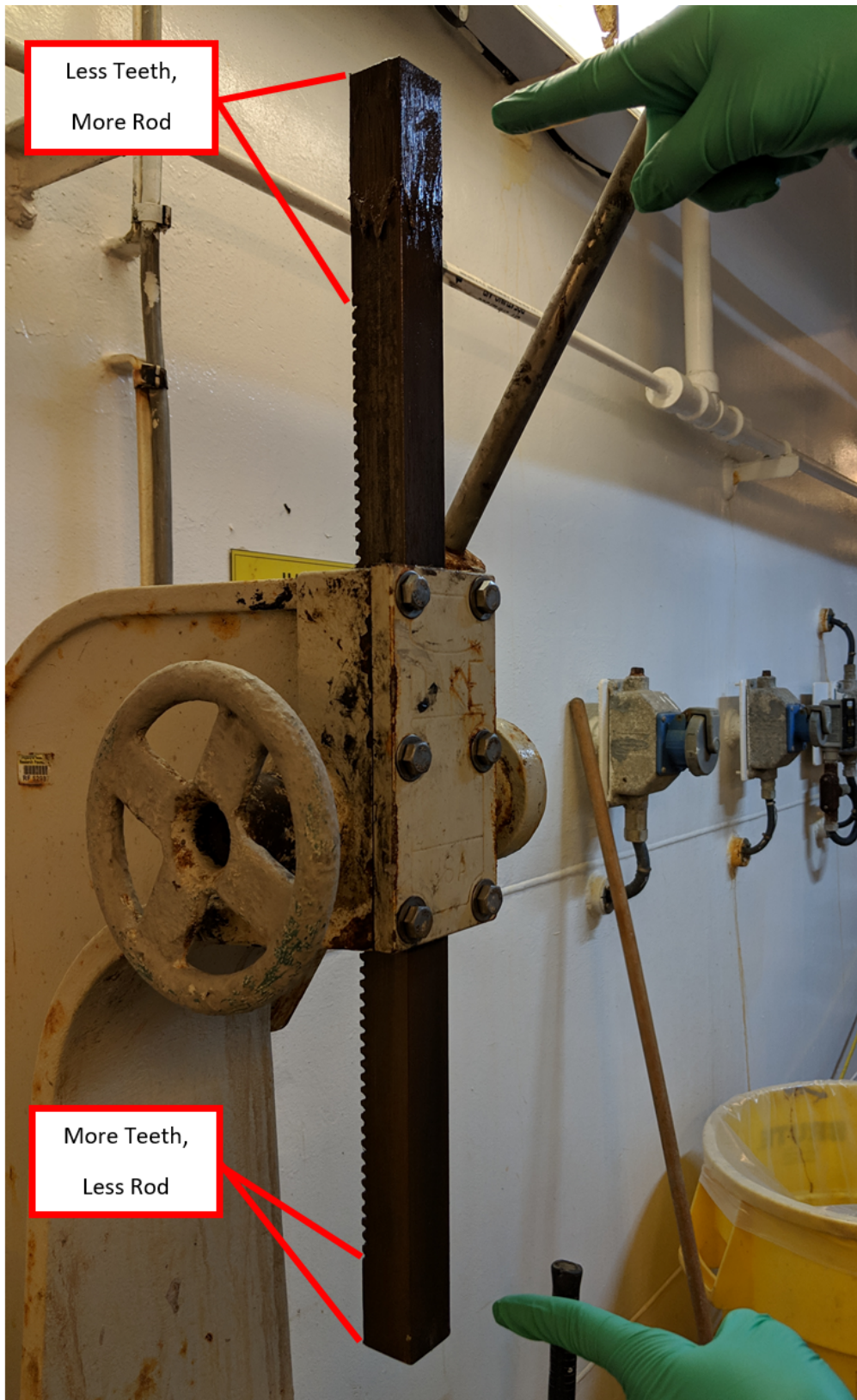
Figure 7: Toothed Square Rod, Proper Configuration
