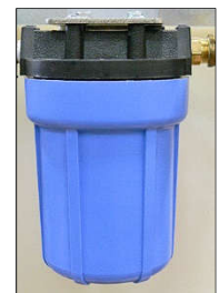
Figure 5-1. Supply Line Filter
