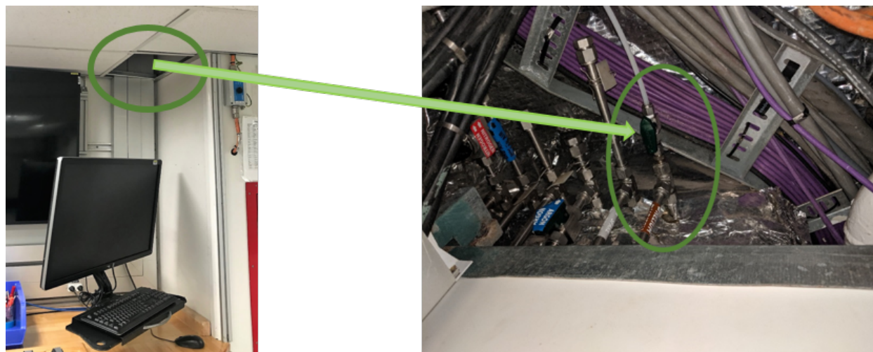
Figure 36. Ceiling panel with He shut-off valve.
