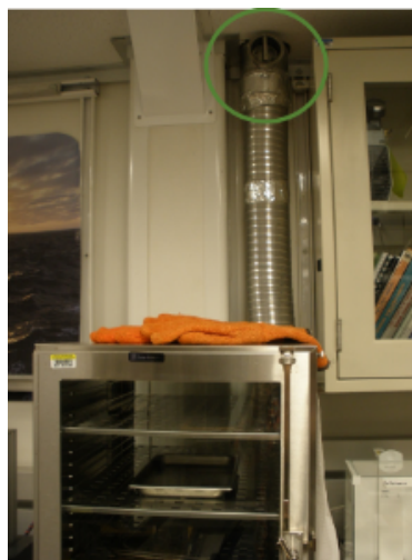
Figure 9. Exhaust tubing and the butterfly valve control (circled in green). The desiccator boxes are to the left of the exhaust tubing.
