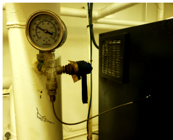
Figure 2: PFMD introduction to mud pump pipeline
