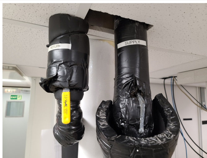
Figure 3: Ship's chill-water valves shown open .
