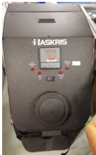
Figure 3: Haskris Water Chiller. This unit is located at the forward end of the paleomagnetism lab. The unit is air cooled and will generate heat in the lab space.
