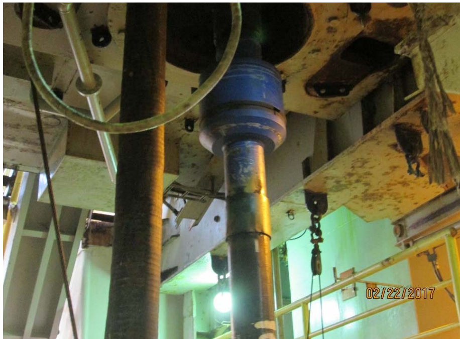
Running in the HRT with Base Adapter connected to 10-3/4" Casing String.
