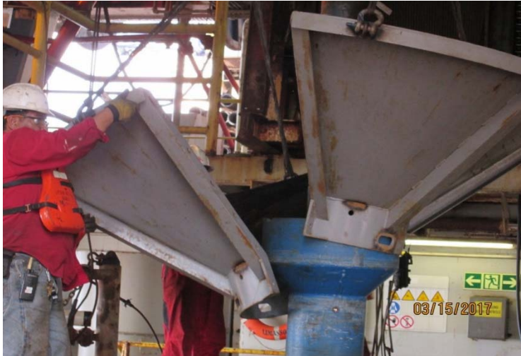
Putting the Re-Entry Cone together in the Moon Pool.
