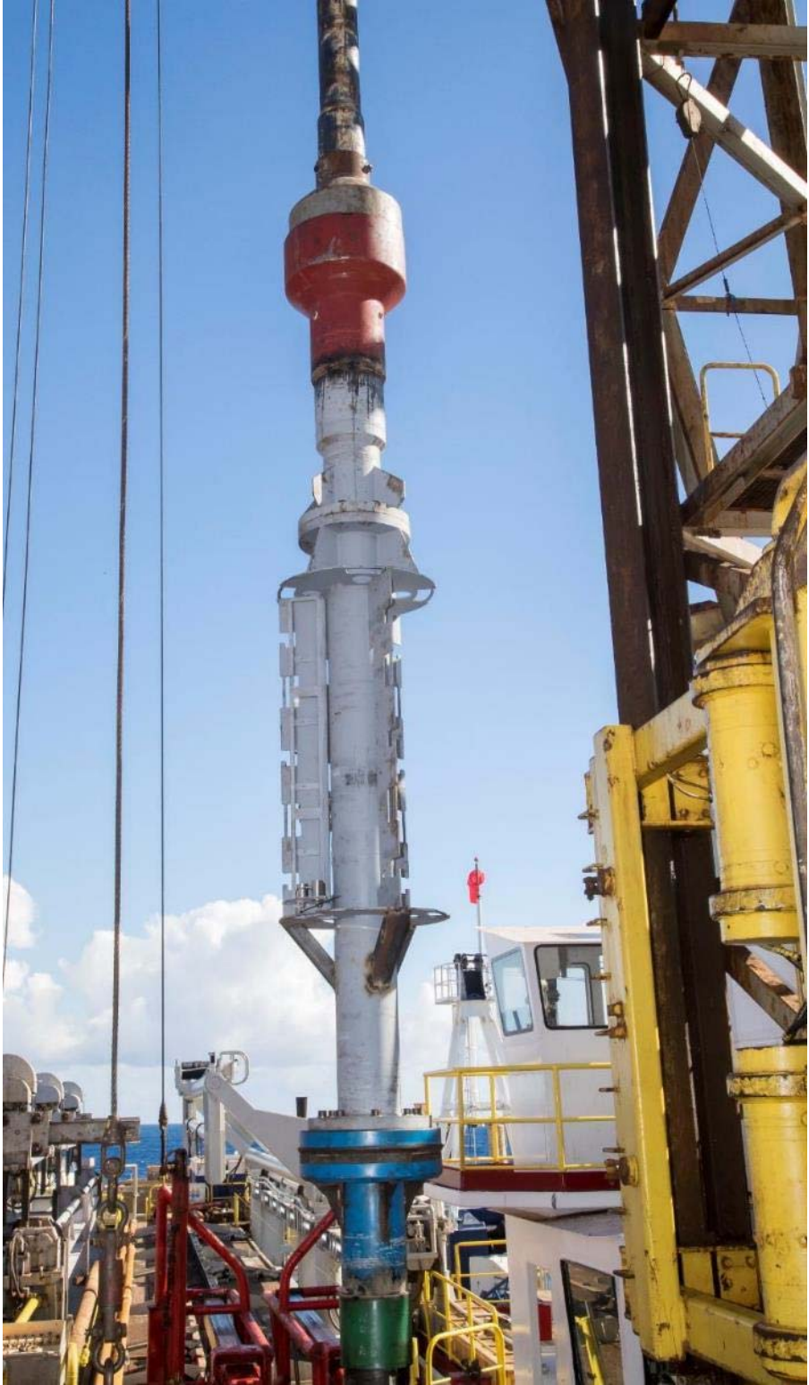
The ACORK in the derrick.
