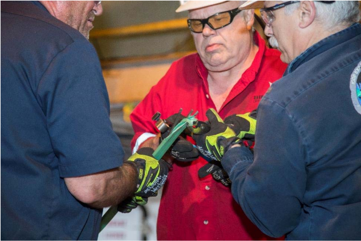
Stripping the armor off the umbilical to make a connection.
