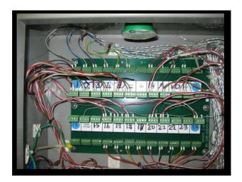
J-BOX to be S/S and be fitted with 12 compression glands to support cable diam of  $\sim 0.33$ " and 1 compression gland for  $\sim 0.8$ " cable.
